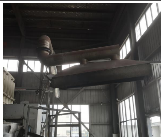
熔化炉烟粉尘废气收集管道及集气罩
